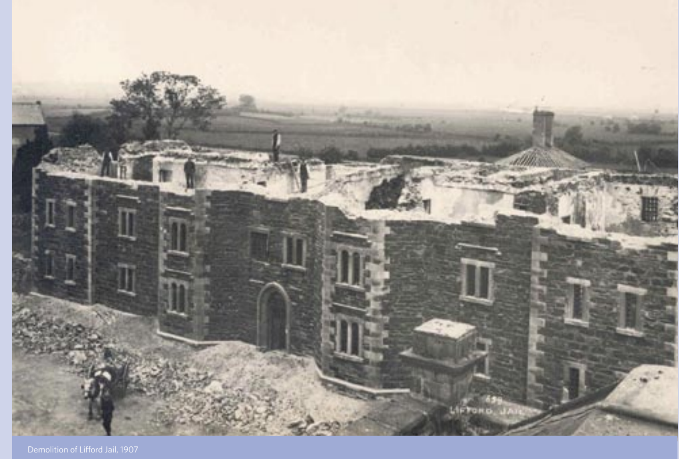
Demolition of Lifford Jail, 1907
