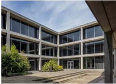
Merrion Hall, Sandymount, designed by Arthur Gibney, Stephenson Gibney & Associates, and completed in 1973. Photo Paul Tierney Photography
