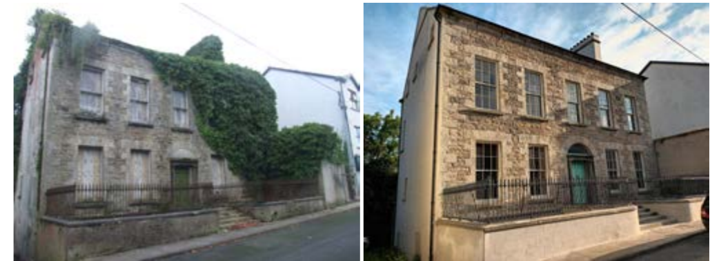
The early nineteenth-century Condon House along The Mall had some of its grandeur restored under the Ballyshannon Historic Towns Initiative. Photo: Donegal County Council
