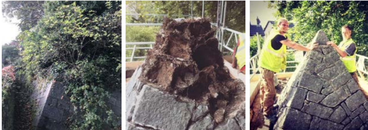
Conservation works on the pyramid mausolea in progress.
