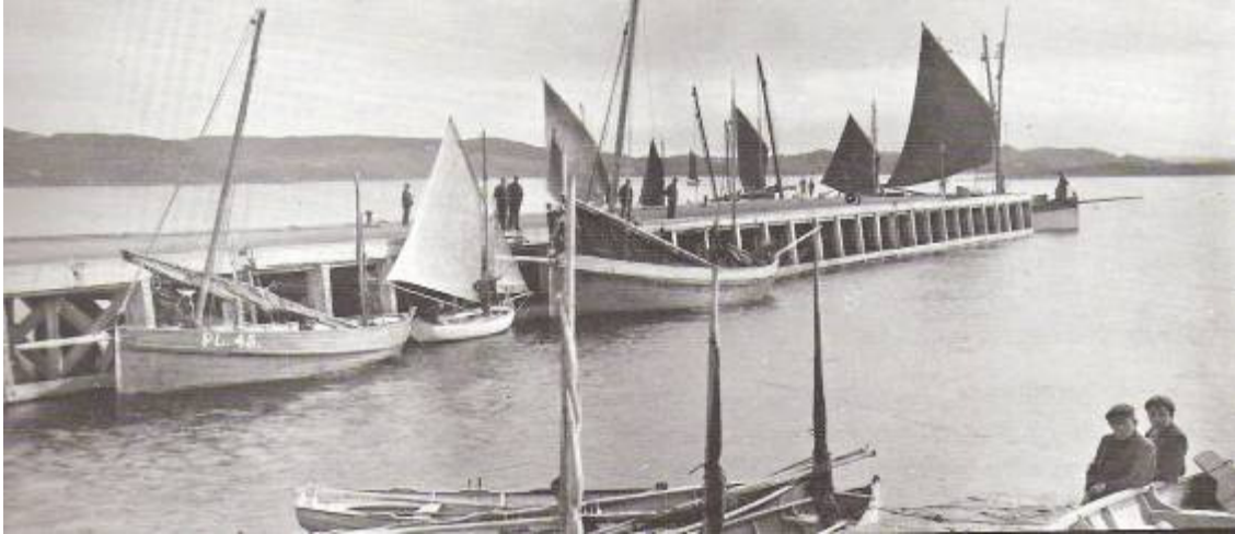
Figure 28: Killybegs wooden pier built by the Congested Districts Board in 1897. This was replaced by a concrete pier in the 1950s. The boats are typical of the period – a ‘nicky’, a ‘nobby’ and in the foreground, three ‘drontheims’ (Photo courtesy of National Museum, Northern Ireland)
