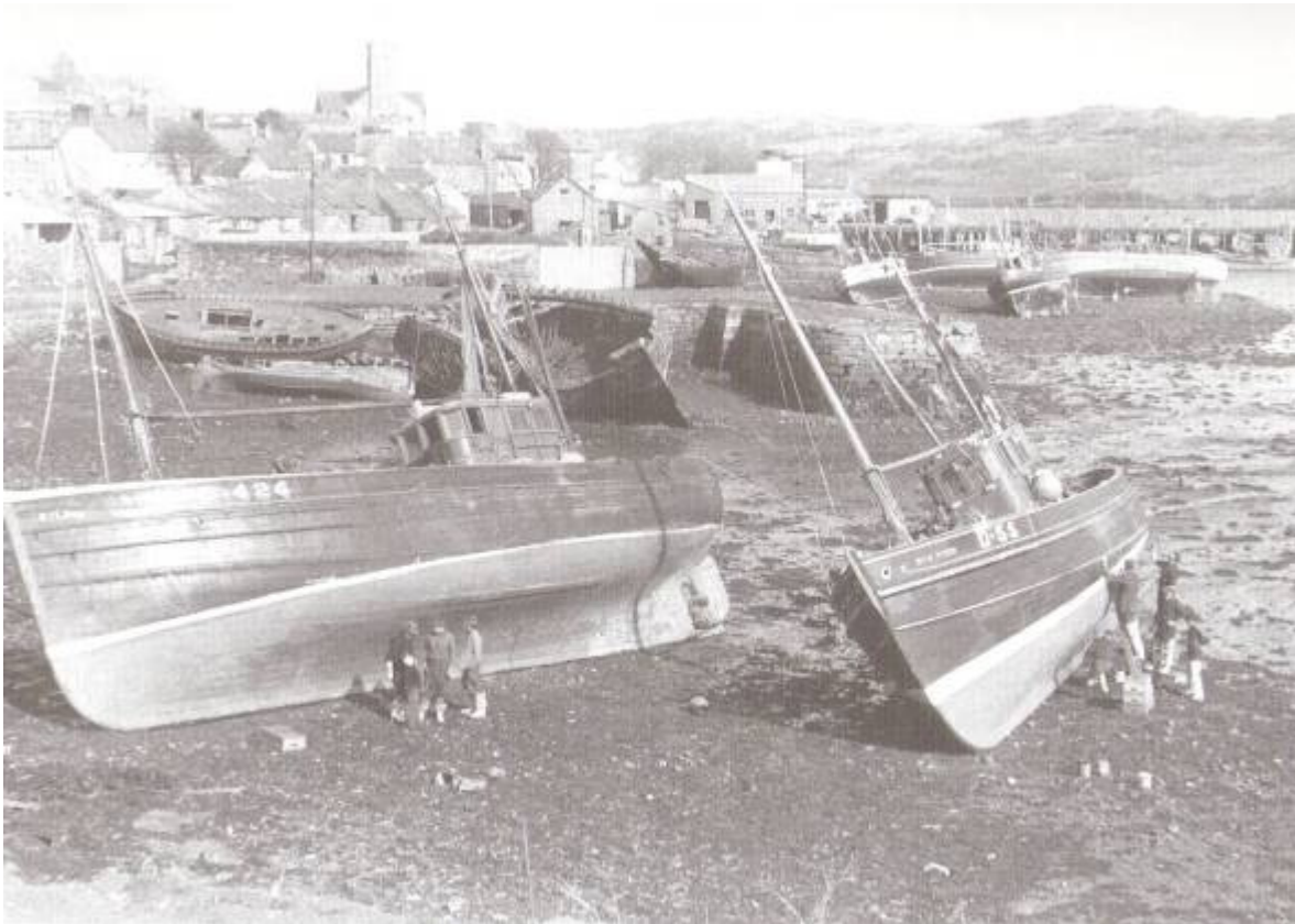
Figure 30: Boats being painted in Kelly's Yard, Killybegs, in 1958
