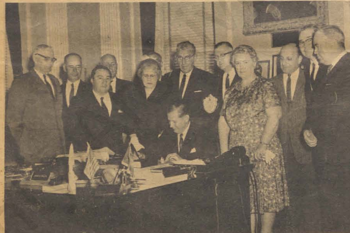
This picture was taken at the State House, Boston, Massachusetts, May 1st, 1962 showing the governor signing the law which made the Foot Bridge on Old Colony Avenue the Hugh Farren Memorial Foot Bridge. On hand for the signing were from left to right: Daniel Doherty, Co-sponsor representing County Donegal and the Central Council of Irish County Clubs, Senator John Powers, Sponsor of the law, Mrs. Helen Doherty, sister of Hugh Farren, Dennis Doherty, husband of Mrs. Helen Doherty, Mrs. Mary McDevatt, County Donegal Clubs.
