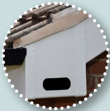
Potential location for nest site entrance in a standard fascia and soffit
