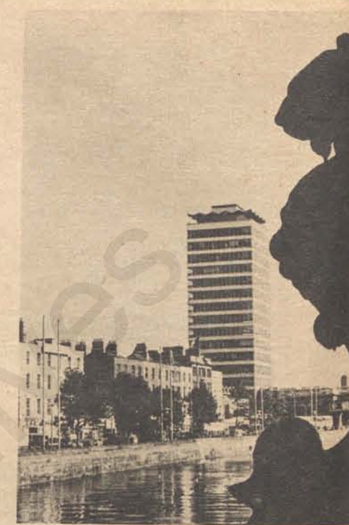
Liberty Hall, 1966, headquarters of the Irish Transport and General Workers' Union and suites of offices, it is Dublin's only skyscraper.
