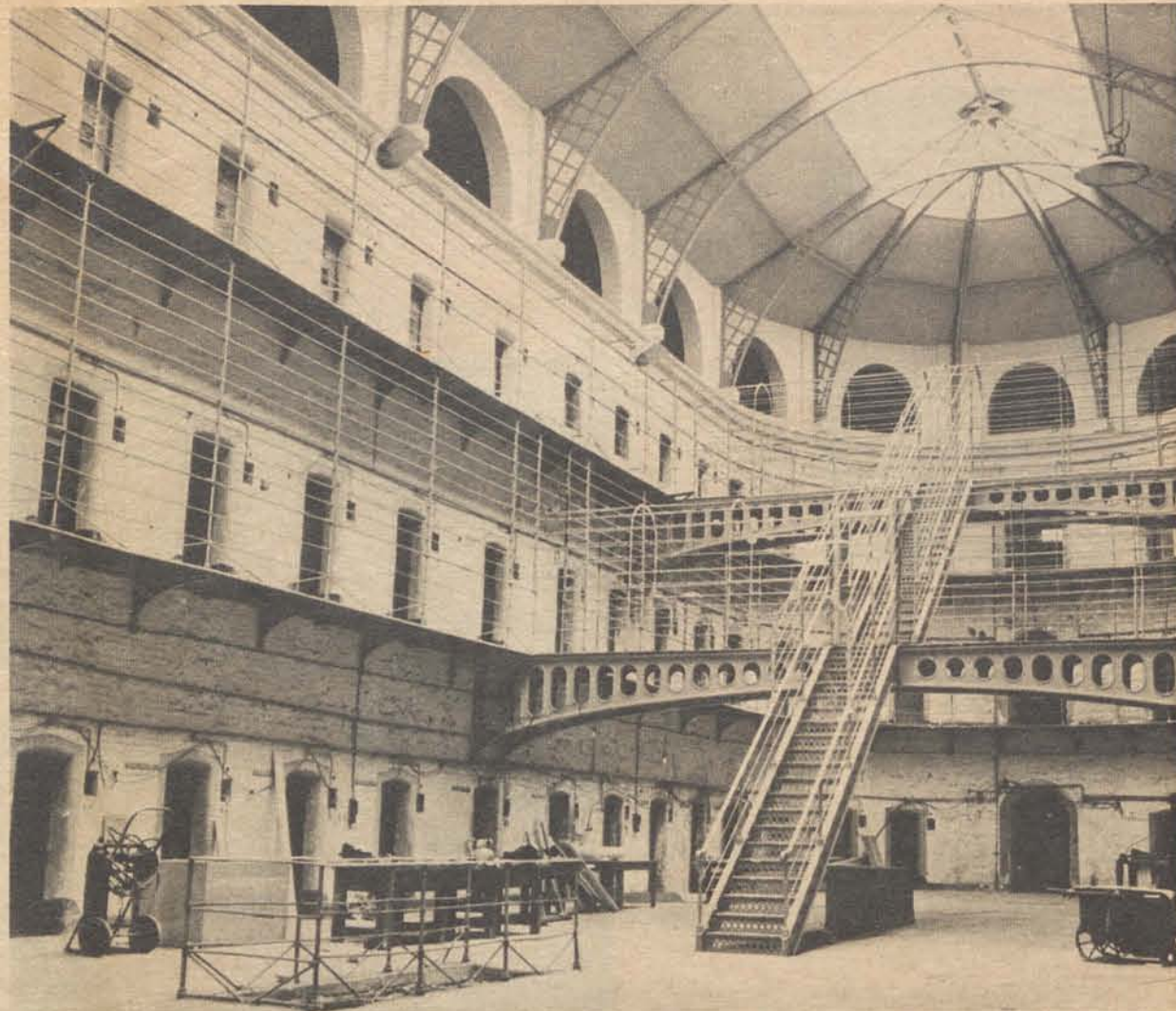
"Interior of Kilmainham Jail. The 1916 leaders were held in the cells on second floor, left."
