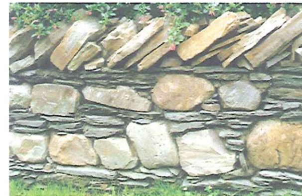
Illust. 17 - A traditionally built stone wall - An Fál Carrach
